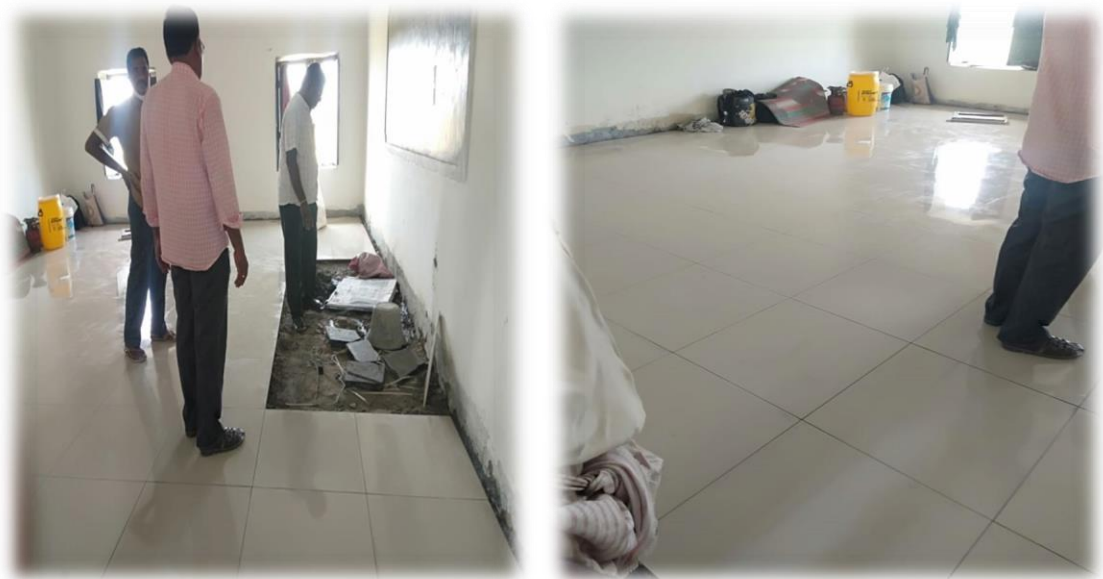
Flooring work of the Class Rooms and Labs in progress with New Tiles
