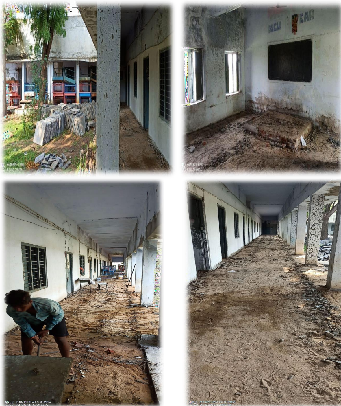
Renovation of Class Rooms and Corridor
