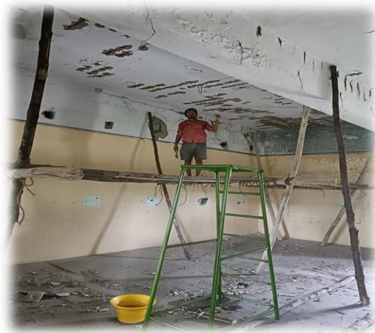
Renovation work going on in the Computer Laboratory
