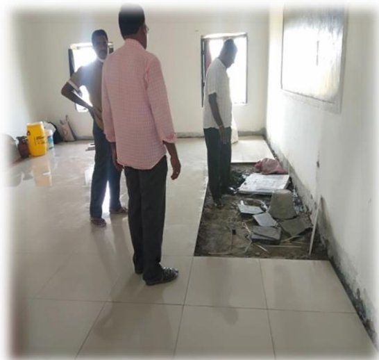
Flooring work of the Class Rooms and Labs in progress with New Tiles
