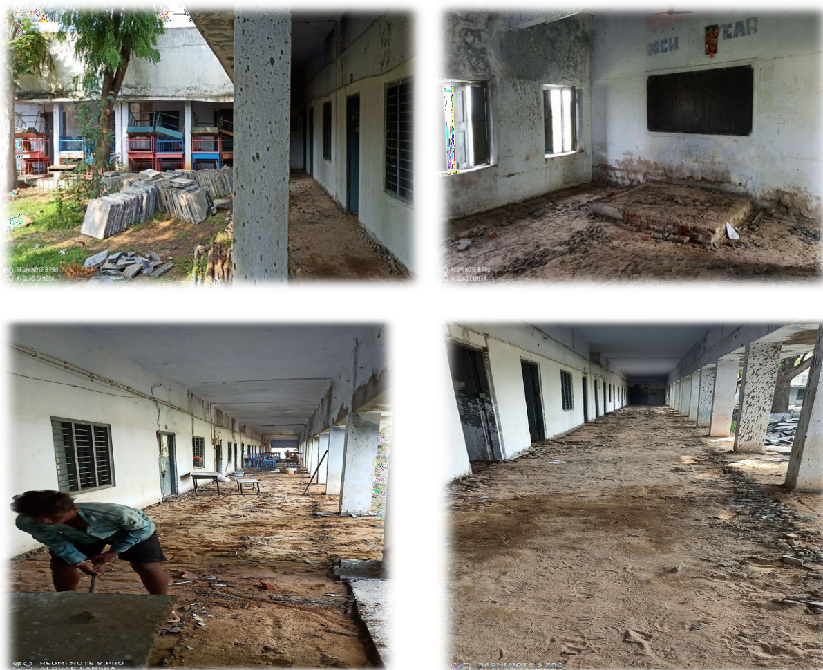
Renovation of Class Rooms and Corridor
